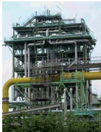
Surveying pipe geometries
