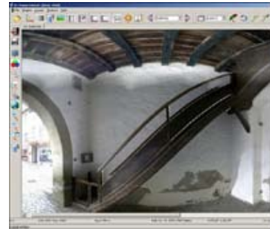
Visualization and evaluation of scan data using Z+F LaserControl. Interior view of Martin's Gate Wangen
